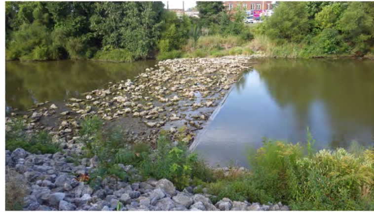
Figure 1 – Blanchard River – Existing Inline Structure - (Cory Street Dam)
