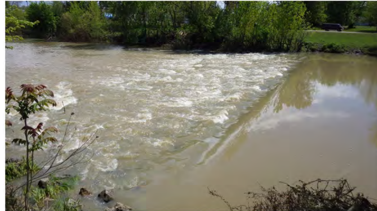
Figure 2 – Blanchard River – Existing Inline Structure - (Centennial Park Dam)
